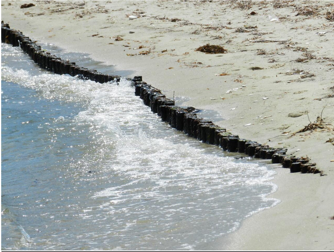
Figure 7.33: Use of the limbs of Pimento trees to arrest beach erosion and promote sand accretion at Placencia and Monkey River
