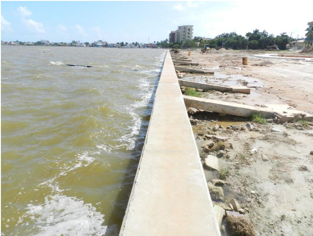
Figure 3.16: Fortified sea wall along the coast of Belize City
